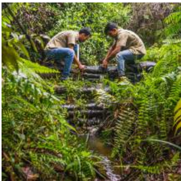
→ Blocking canals using sand bags
